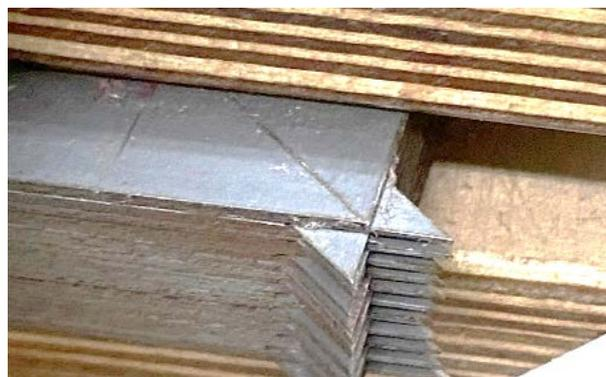
Figure 8. Iron core overlap area
